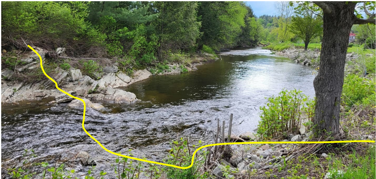
Figure 4: Confined Bedrock Channel Section 420 Feet Downstream of Williams Dam (Looking Downstream)
